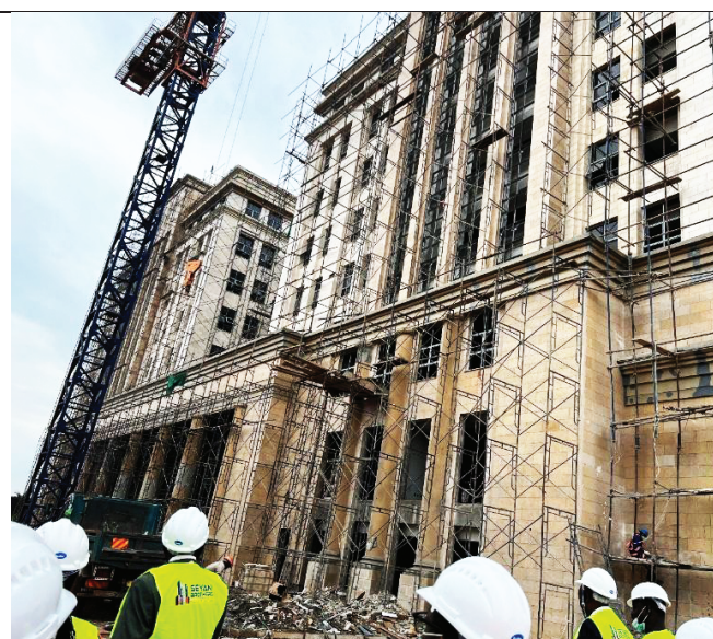
Status of the construction
